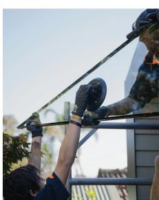
and failed to come up with a solution; Rob and the Glass Express team were confident they could organise an aquarium to relocate the fish to a temporary tank, drain the water, remove slip hazards, crane the glass panel in using a suction cups and a 350 kg counter weight (without damaging the house), install and silicone the new glass window into place, refill the pond, and return the fish! The customer was overjoyed with the end result' beams Rob.
